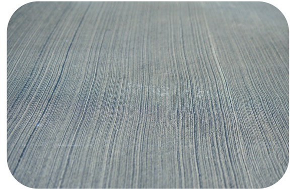
A nonslip concrete surface
